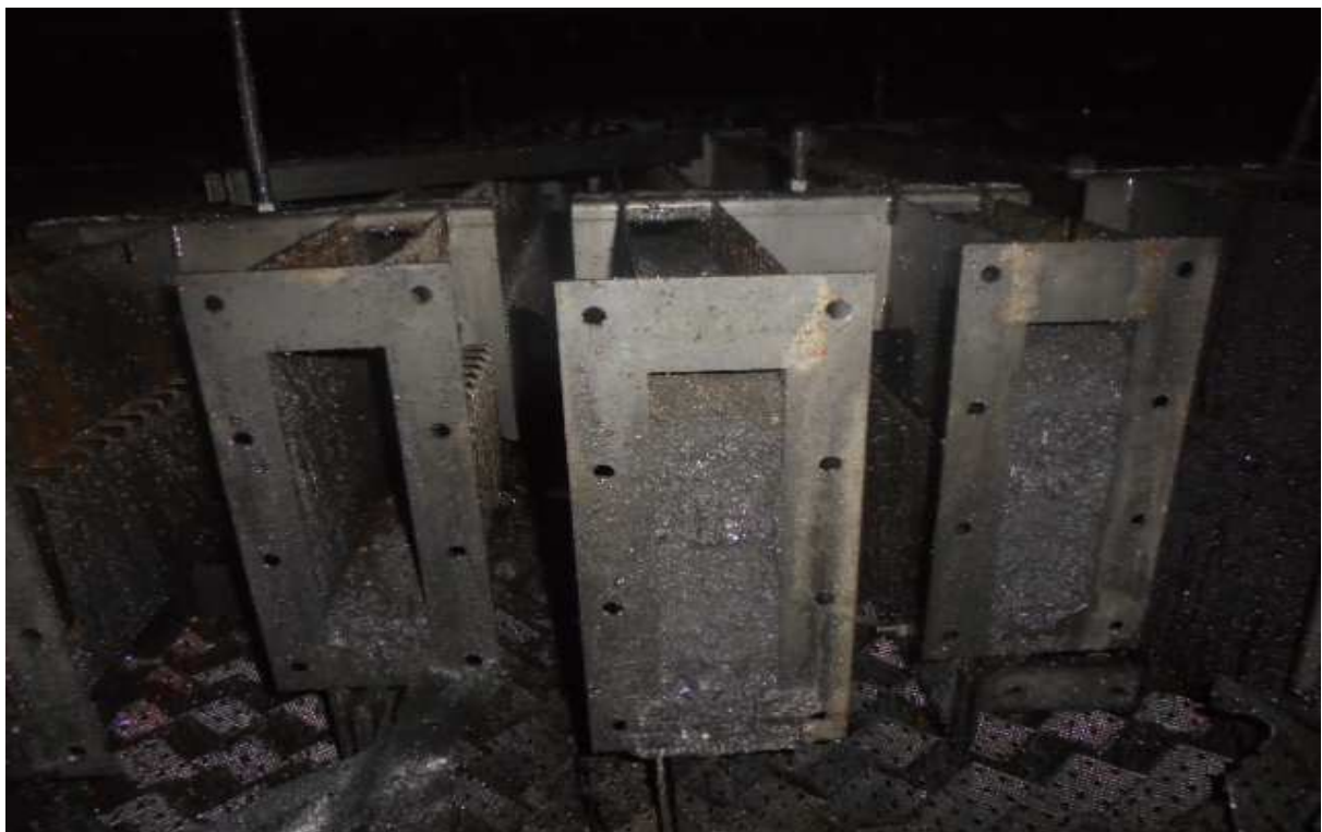
Figure 5: Plugged trough distributor
